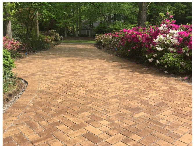
Newly installed permeable pavement. Photograph by Robyn Woolsey.
